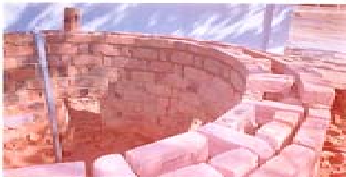
Figure 2c. Kiln wall during construction
