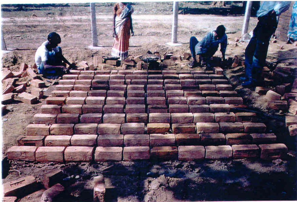
Figure 3: Kiln floor during construction
