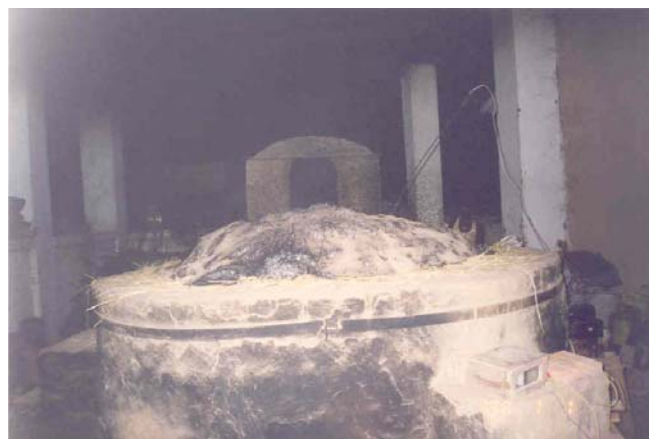
Figure 5: Belt to improve structural strength of kiln
